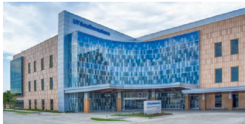
UT Southwestern Monty and Tex Moncrief Medical Center at Fort Worth
